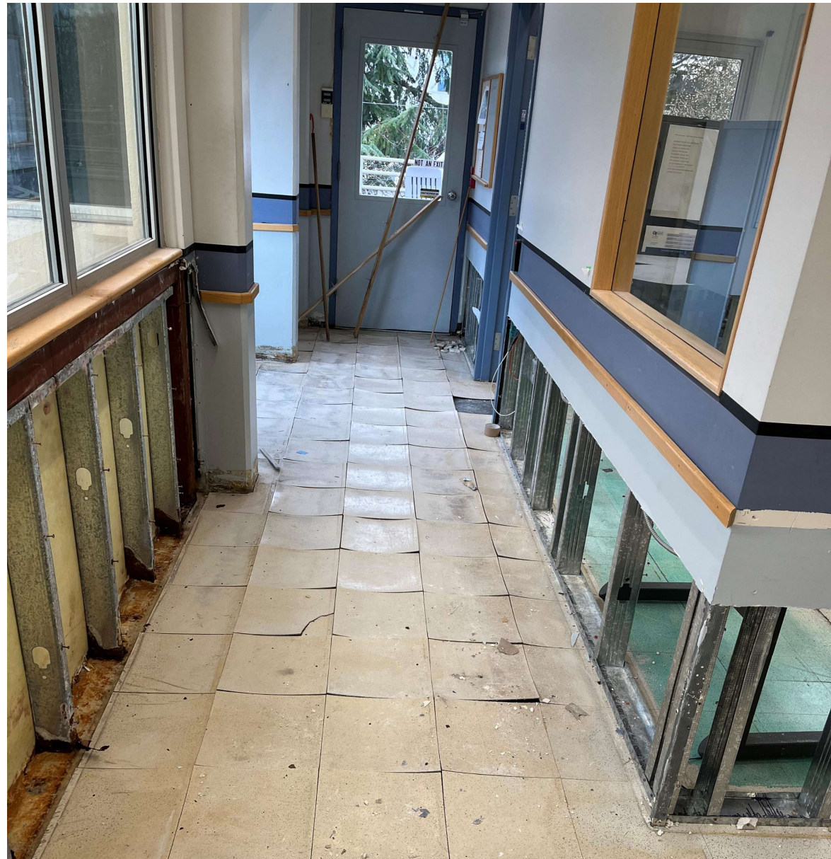
WTP 2 nd FLOOR AFTER INITIAL DEOMOLITION
